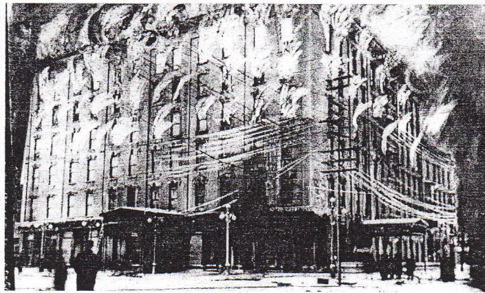
On the night of February 6, 1912 the Hotel Downey was destroyed by fire, losses were estimated at $109,991. The hotel was expanded in 1907-1910 when two stories were added to the structure and the new sixth floor became a convention hall. After the fire the building was quickly rebuilt because none of the exterior walls of the building were damaged in the fire.
